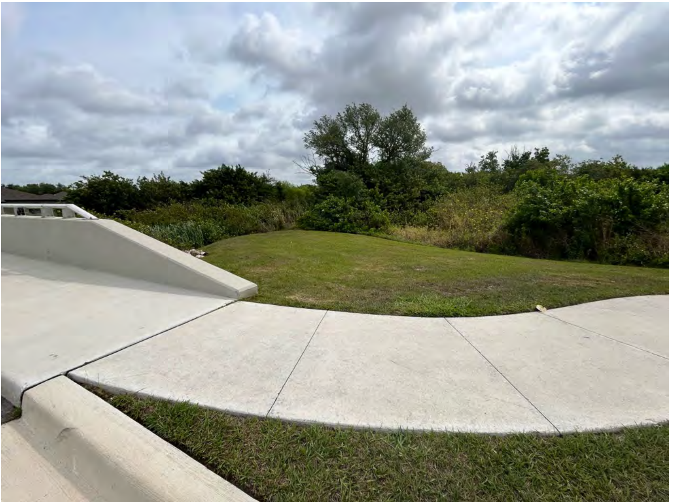
Bridge Area- Mowed and Line Trimmed
